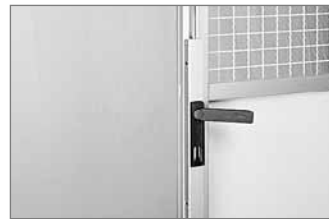
Lock mechanism for double door (p. 10-17)
